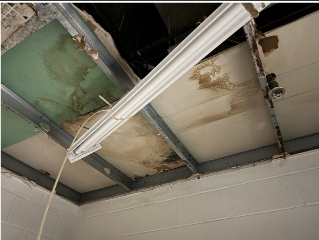
Water damage and mold visibly present in storage room area
